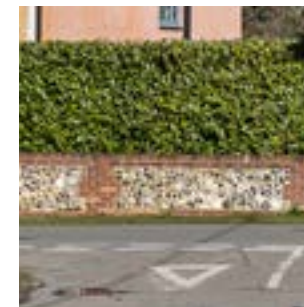
Brick and stone low wall
