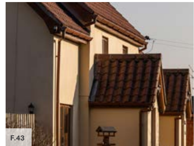
Figure 43: Contemporary dwellings using local traditional materials and roof elements (gabled porches) (credit: Peter Leonard)
