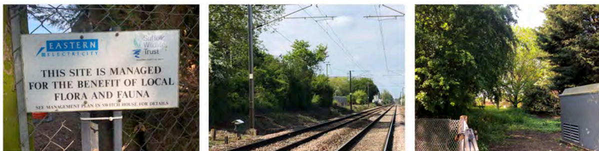
Figure 67 all: Hales Street nature reserve UK Power Networks Tivetshall Primary substation.
